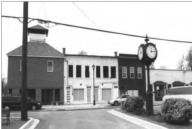
Historic core: Mix of heights, from approximately 14 to 28 feet, one story or two.
