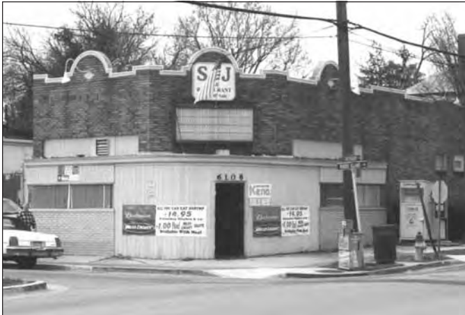
Renovations mask the building's original entrance on the corner and its architectural detailing.
