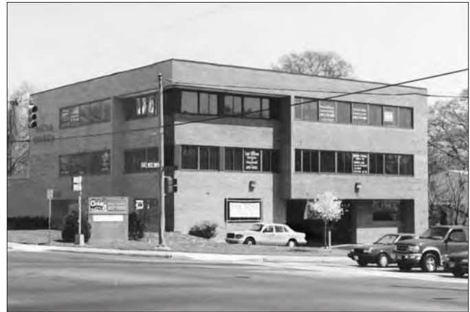
Horizontal window banding, a distinctive characteristic of late twentieth-century office buildings.
